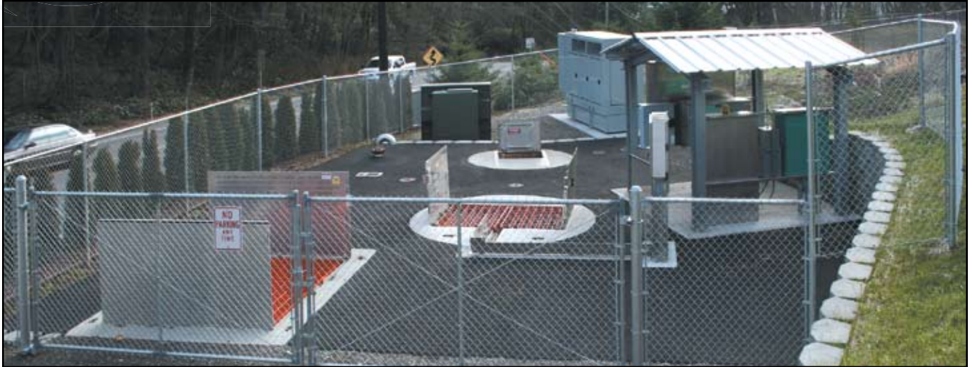
New Romtec Utilities wastewater lift station.
