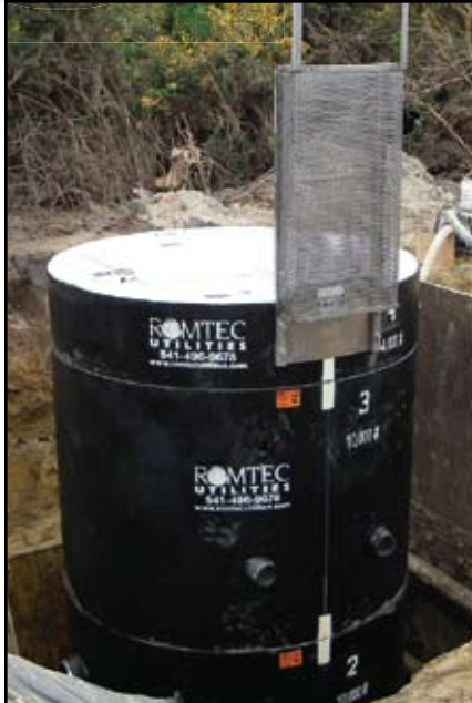
New wet well with Tnemec coating.
