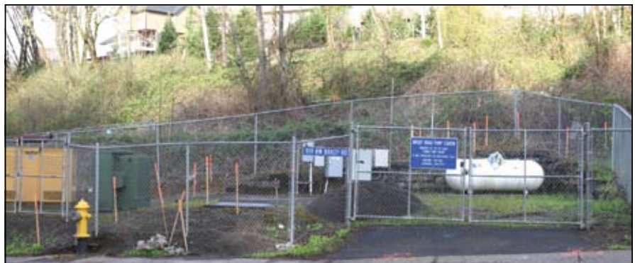
Old pump station before replacement.
