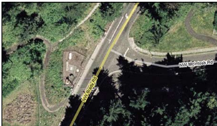
Aerial view of old pump station at intersection of NW Brady Rd and McIntosh Rd.
