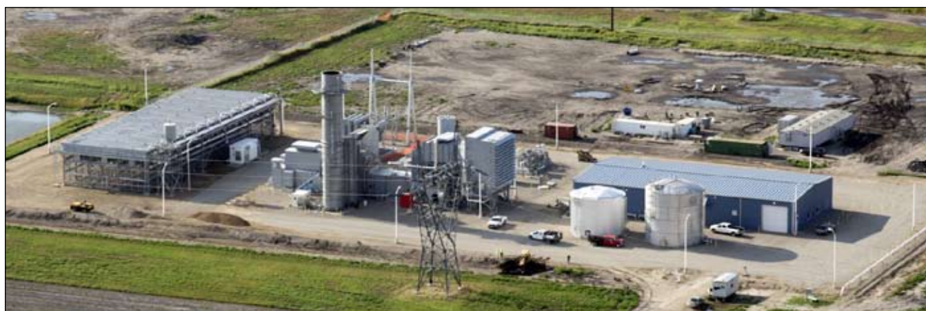
A second generator would soon join the world's first commercial GE Energy LMS100. (2006 photo courtesy of BEPC)
