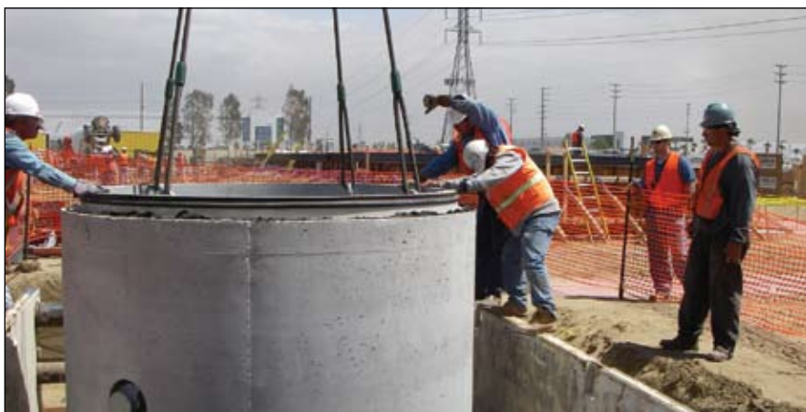
Workers lower a wet well barrel section into place.
