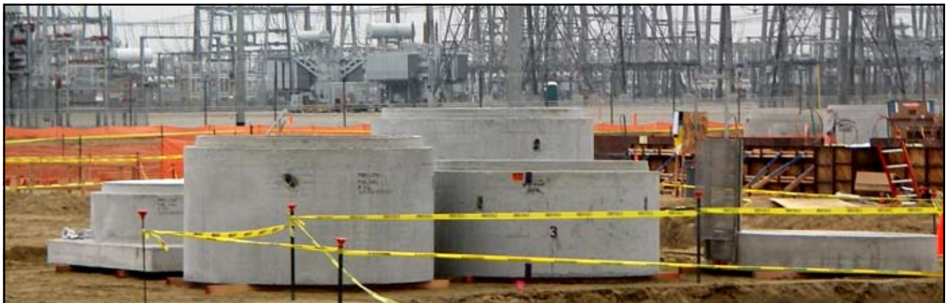
Wet well, delivered to site, awaits installation.
