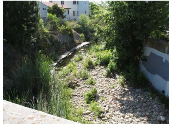
Mission Creek viewed from Haley Street Bridge
