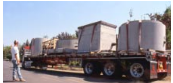
Complete lift station arrives at job site in a single delivery.
