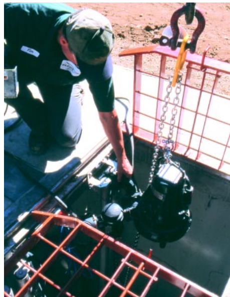
(this photo) Romtec Utilities Top Slab with Flygt Safe-Hatch and Pump Disconnect Panel & Stand (below) Flygt technician uses guide rails to lower submersible pump into wet well through half-open hatch.
