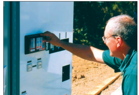
An ITT Flygt technician programs the MultiTrode controller during start-up of a Romtec lift station.
