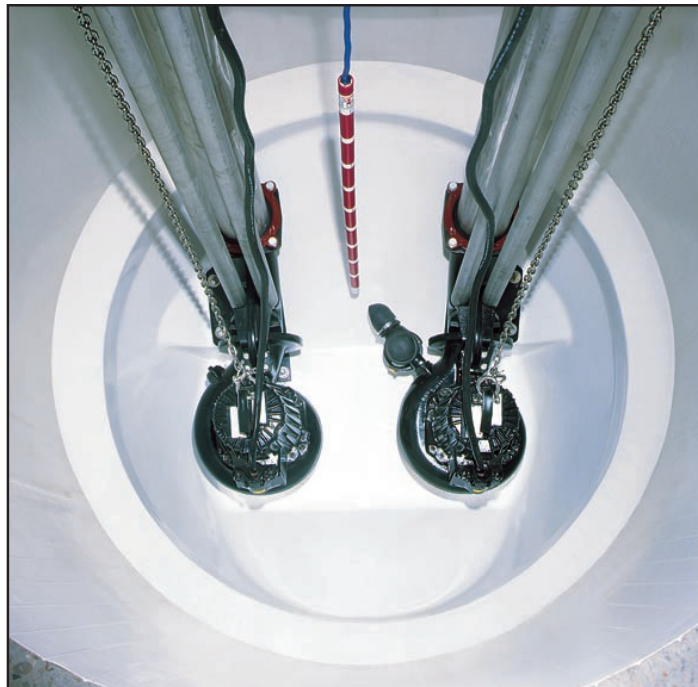
The MultiTrode conductive level sensing probe is suspended between two submersible pumps.
