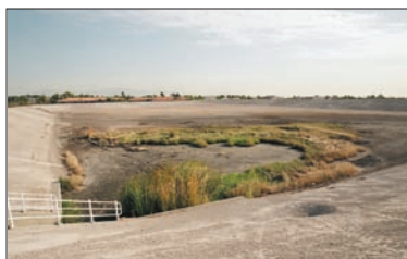
The lift station drains the 10-acre Desert Inn Detention Basin in Las Vegas, Nev.
