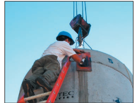
Romtec Utilities' Pre-Engineered Package Lift Stations include self-cleaning, pre-cast concrete wet wells in 6- and 8-foot diameters. The base, barrels and top slab are pre-aligned for ease of installation.
