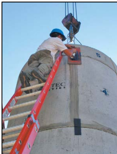
Alignment marks are painted on the barrel sections for easy installation of the wet well’s barrel sections. The new 8-foot wet well is nationally shippable, and comes to the job site ready to be installed by crane.
