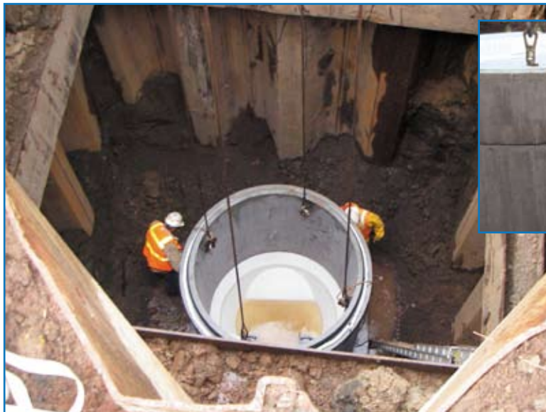
Construction workers check the wet well base at Lacamas Meadows. Top, alignment marks on the wet well barrel sections and top slab ensure accurate installation.
