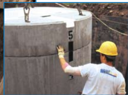
Construction workers check the wet well base at Lacamas Meadows. Top, alignment marks on the wet well barrel sections and top slab ensure accurate installation.
