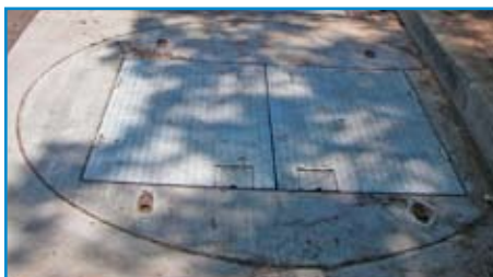
The lift station control panel and electrical controls sit just off busy Haley St. in downtown Santa Barbara, Calif., while the wet well and valve vault are actually placed in the street (below).
