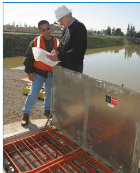
Frank Quach, project inspector of Mark Thomas & Co., and Bob McLean of Shape Inc., review a lift station drawing next to the large detention pond in Union City, Calif. The Romtec Utilities wet well (foreground) is equipped with two Flygt submersible pumps for draining the pond after storms.
