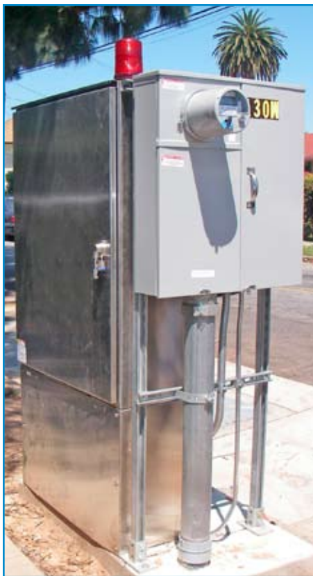
The lift station control panel and electrical controls sit just off busy Haley St. in downtown Santa Barbara, Calif., while the wet well and valve vault are actually placed in the street (below).
