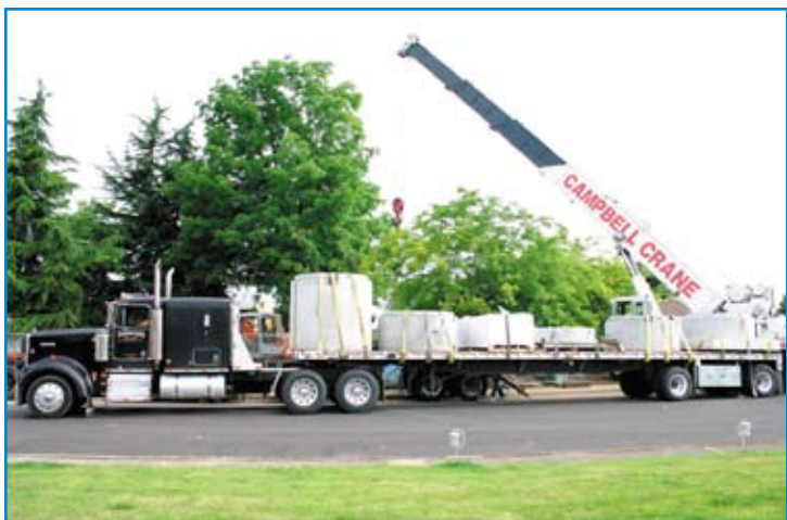
Romtec Utilities lift stations arrive in a single delivery, making most efficient use of crane service.
