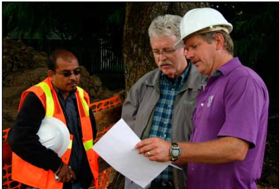
Romtec's Jim Baird discusses the Woodburn wet well installation with public works and engineering staff.
