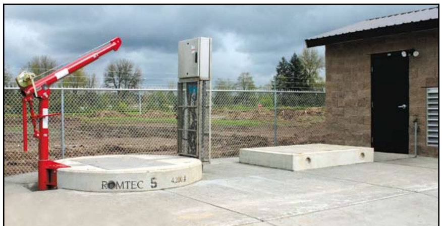
Bottom: Romtec Utilities lift station includes: wet well with Flygt submersible pumps, Thern crane and pump disconnect panel; valve vault with pre-assembled valves; building with station control panel, Cummins generator with automatic transfer switch and air injection system.
