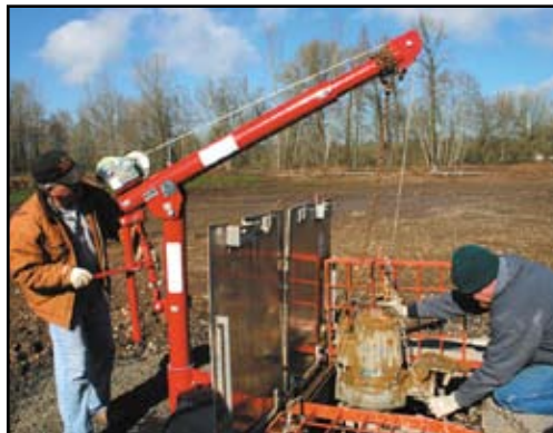
Far Left: Double steel doors provide access to the Cummins standby generator with QuietSite II sound attenuation enclosure.
