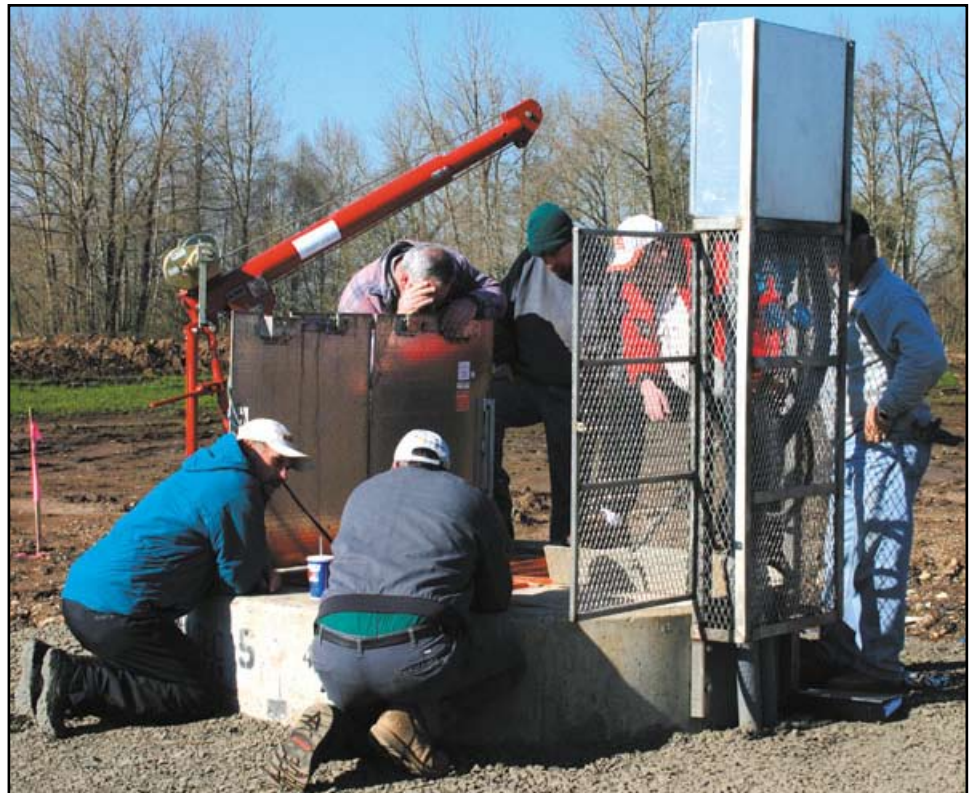
City officials, contractors and technicians inspect the new wet well.
