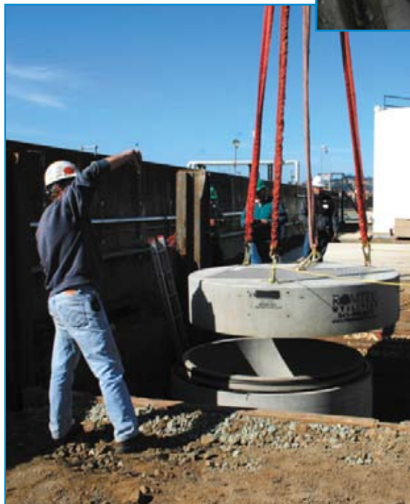
Final wet well section is pre-cast top slab with access hatch.
