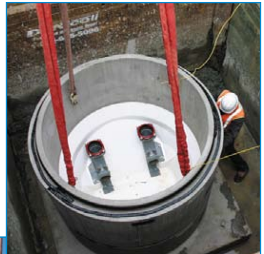
Second section of wet well is placed on base.
